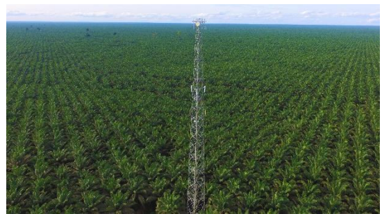
Mobile telecommunications tower
