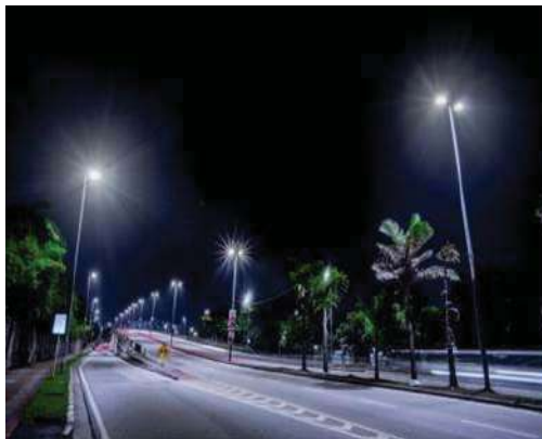
LED street lights
