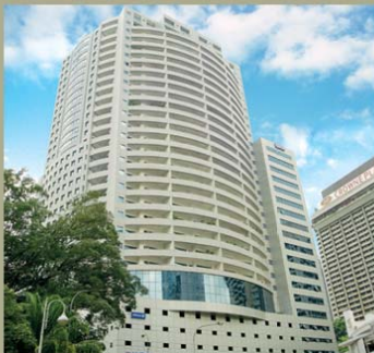
WISMA UOA CENTRE
