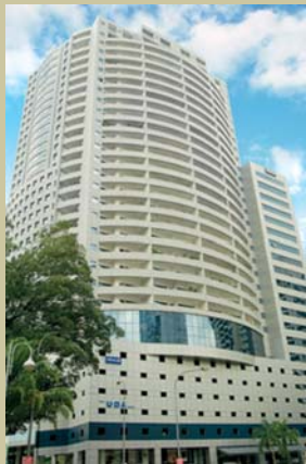
WISMA UOA CENTRE
