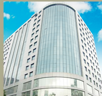
WISMA UOA DAMANSARA
