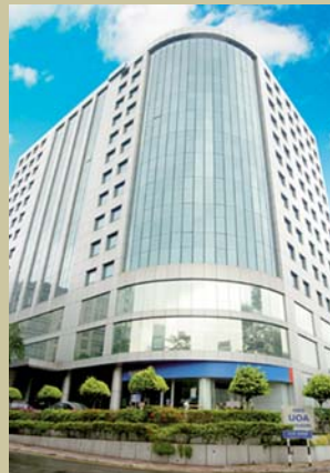
WISMA UOA DAMANSARA
