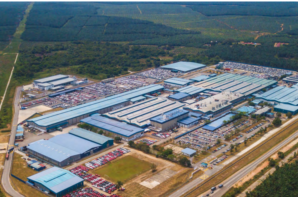
Inokom has embarked on a company-wide initiative to improve energy efficiency at their assembly plant in Kulim, Kedah.
