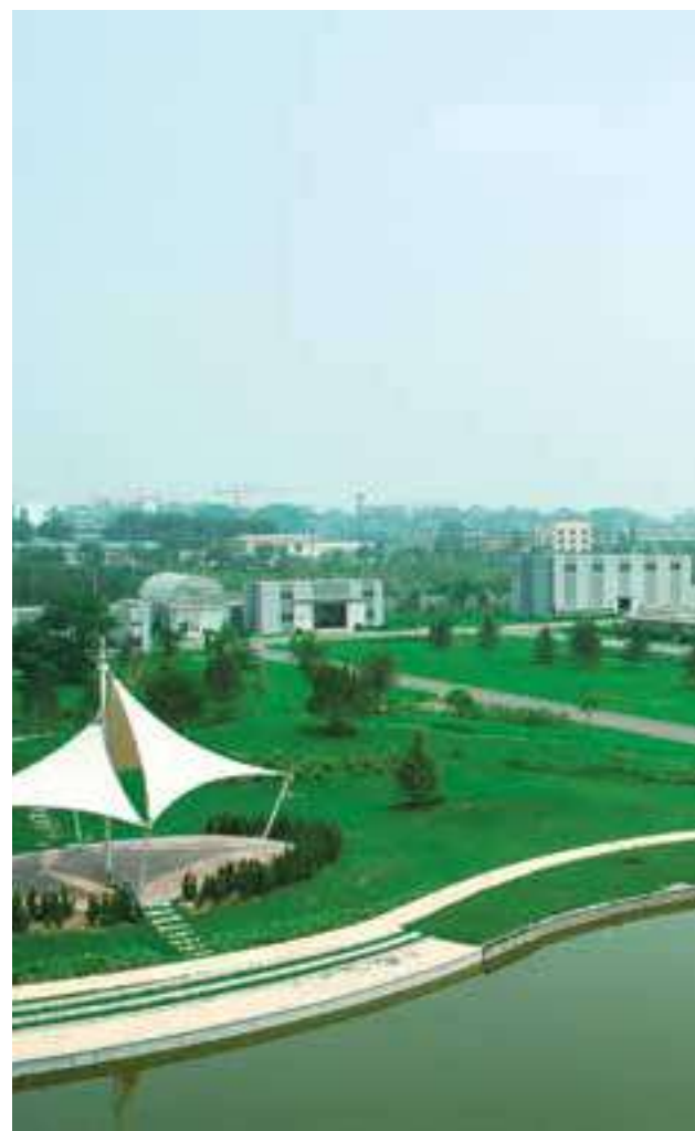
Lugouqiao Sewage Treatment Plant in Beijing, China
