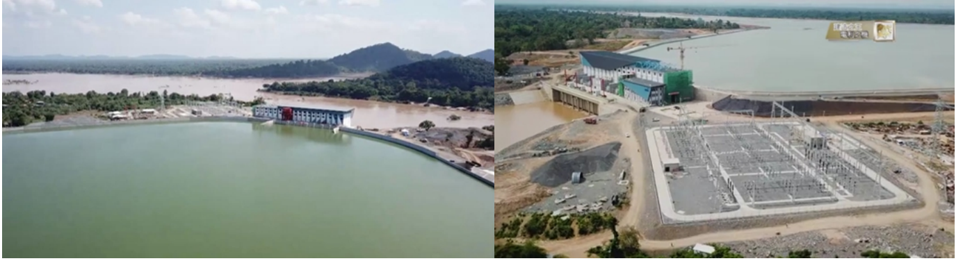
Figure 3: Aerial View of 260MW- Don Sahong Hydropower Project, Laos (92.1% completed)
