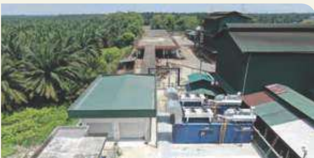
Power Plant Facilities
