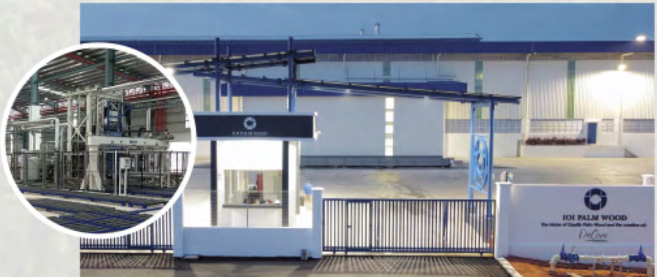
IOI's new Palm Wood Manufacturing facility in Johor
