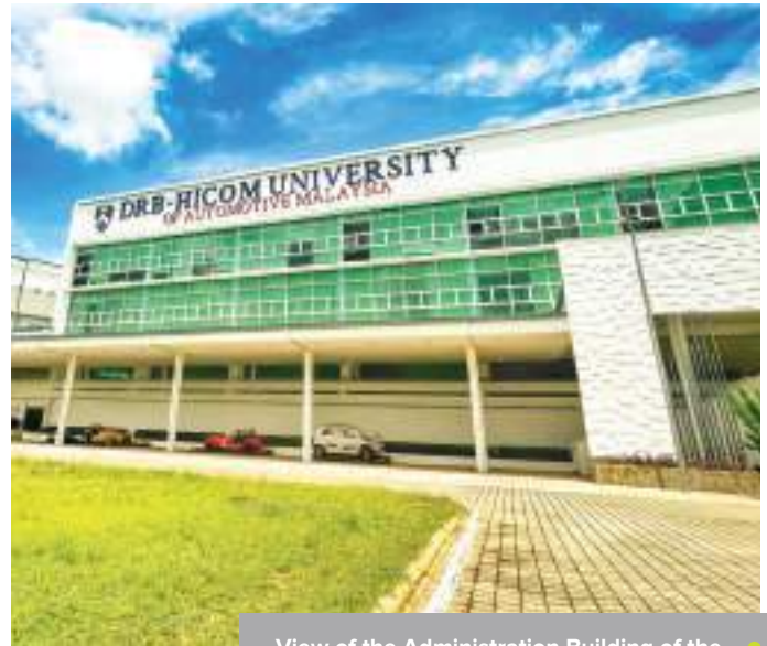
View of the Administration Building of the DRB-HICOM University in Pekan
