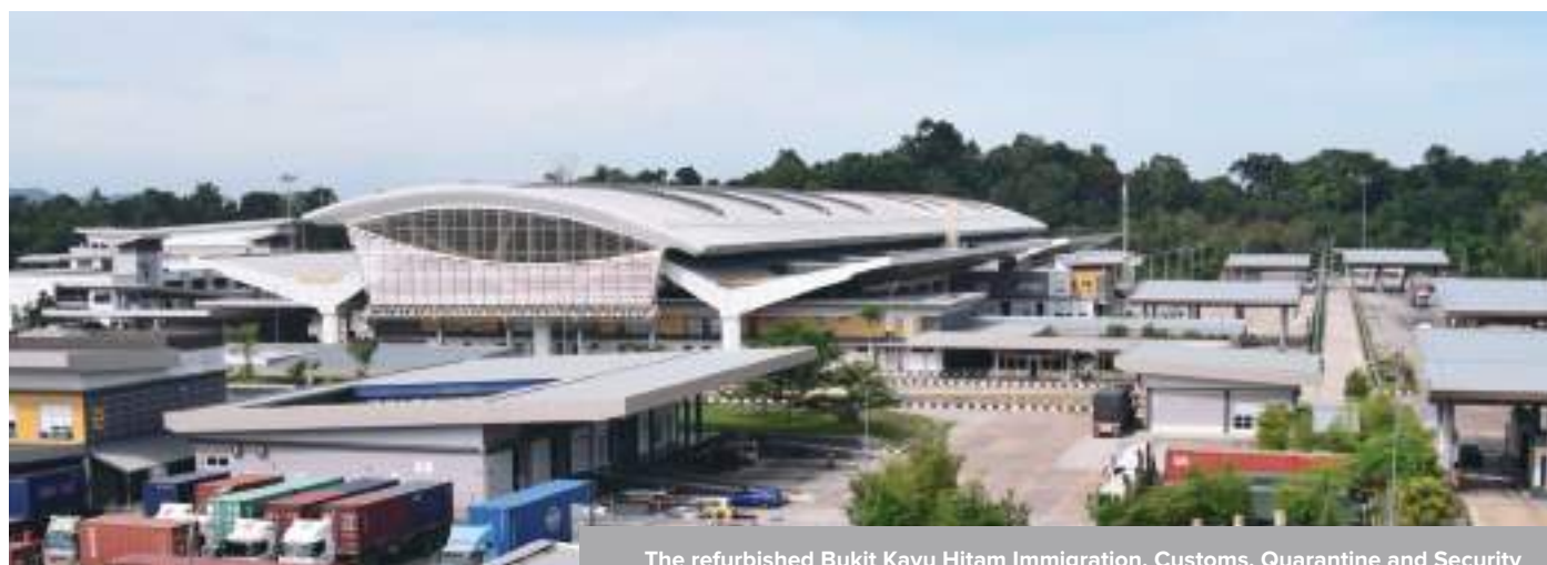
The refurbished Bukit Kayu Hitam Immigration, Customs, Quarantine and Security Complex in Kedah has made the border-crossing process significantly more efficient
