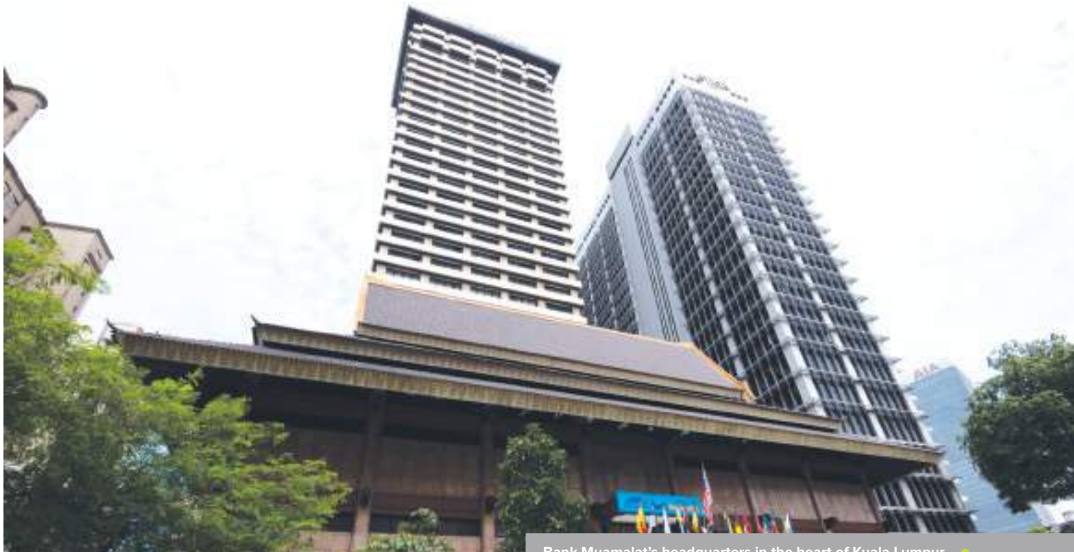
Bank Muamalat's headquarters in the heart of Kuala Lumpur
