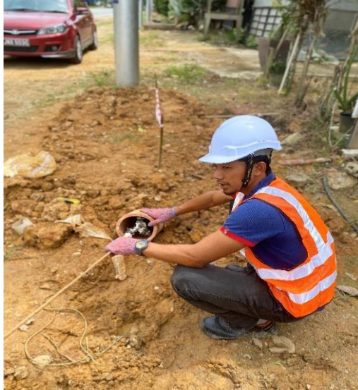
Tracing officers pulling the gyroscopic surveying tool from HDD exit pit
