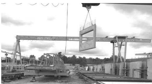
Removal of formwork (i.e. IBS component) for storage
