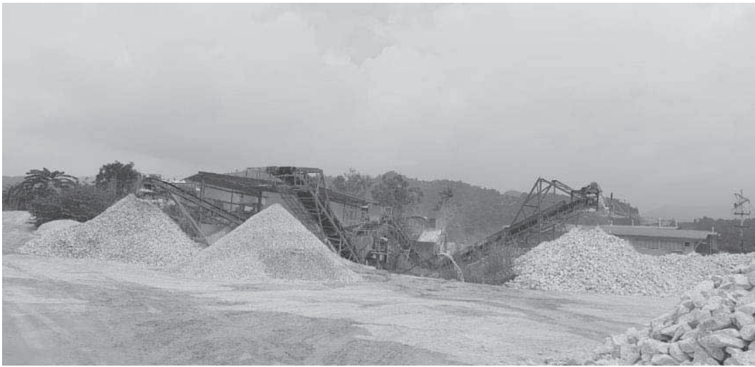
Our contractor's primary crushing plant at Perak Quarry 1
