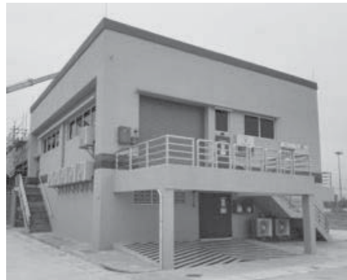
33kV substation for a medical device manufacturing plant
