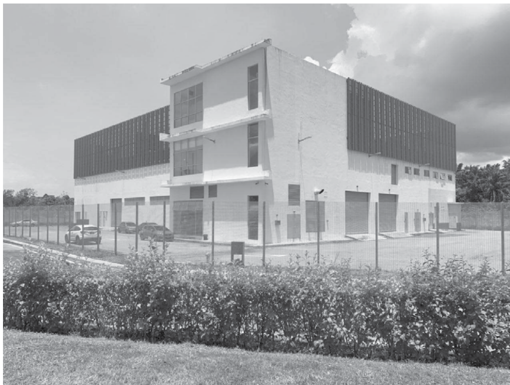
A district cooling plant
