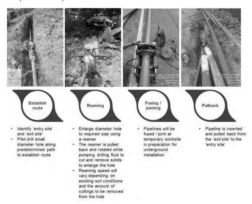
This method is suitable for laying power cables, telecommunication cables, fibre optic cables and gas pipes. HDD is a method to avoid natural (such as rivers and forests) and man-made objects (such as roadways, railways and building structures) when connecting utility pipelines to minimise the impact on the area above the drilling route.
