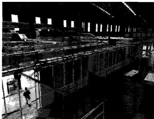
Class 10,000 ISO 7 cleanroom project for a semiconductor manufacturing facility in Batu Kawan Industrial Park, Pulau Pinang
