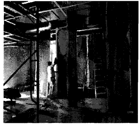
Wall panel installation
