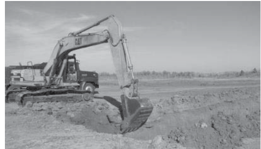
Site clearance and earthworks
