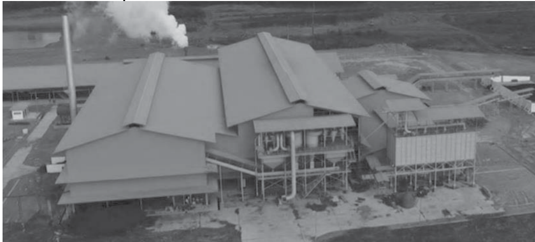
The palm oil mill we constructed at Mouila Plantation in Gabon
