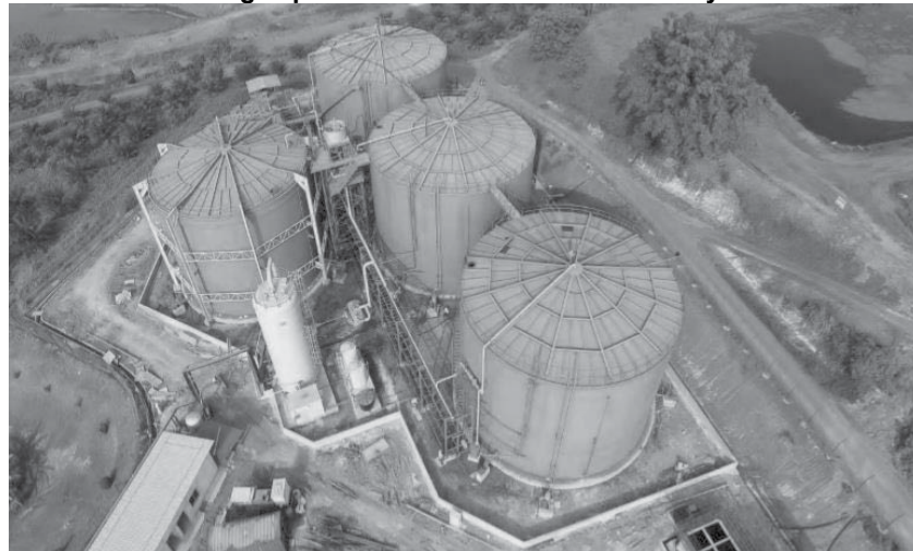
A biogas plant that we constructed in Malaysia
