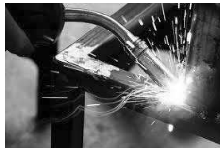
MIG welding process
