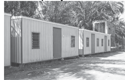
Temporary Site Office
