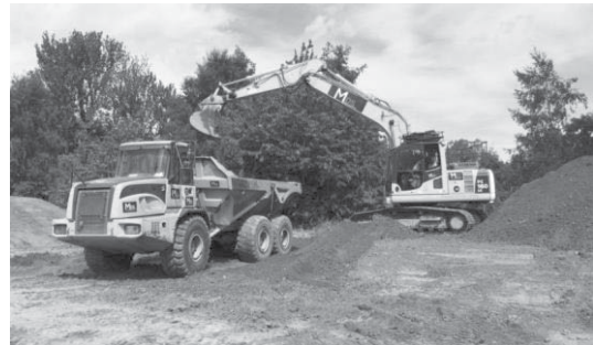
Site clearance and earthworks
