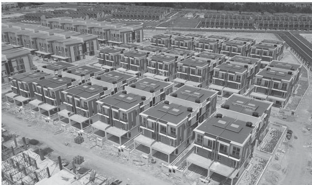
30 TSSD Taman Nusa Sentral Project
