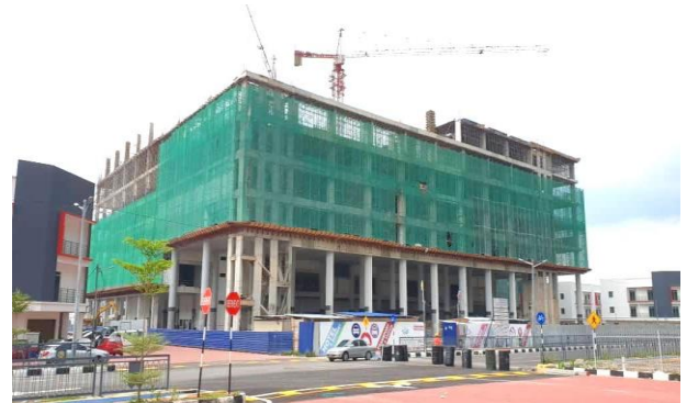
Fig 2: Site progress at Kampar Terminal
