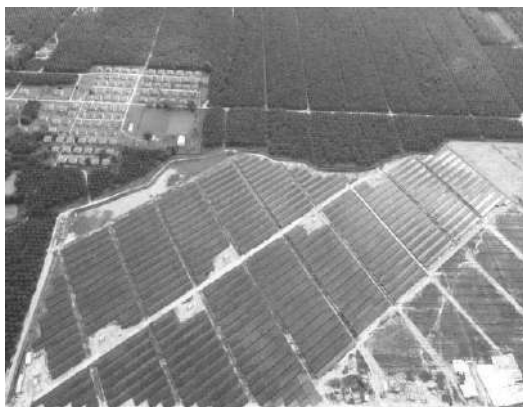
Aerial view of an LSSPV plant
