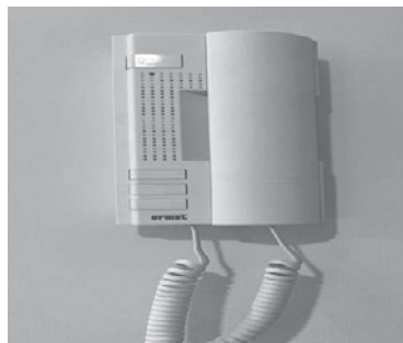
In-building telephone system
