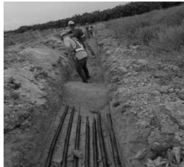
Earthing works and cable laying works
