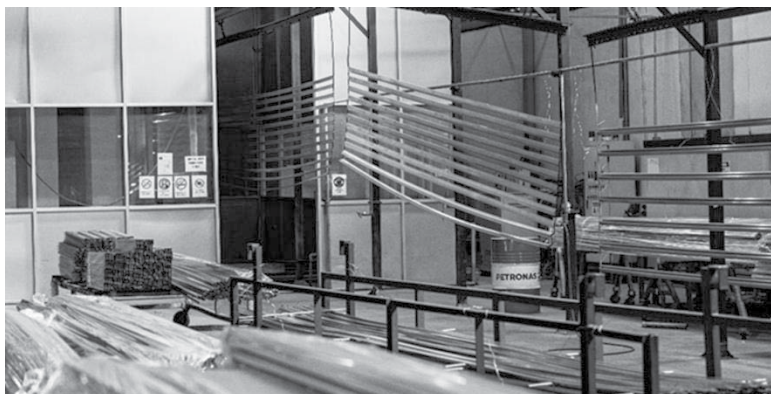
Extruded aluminium profiles entering the automated powder coating room
